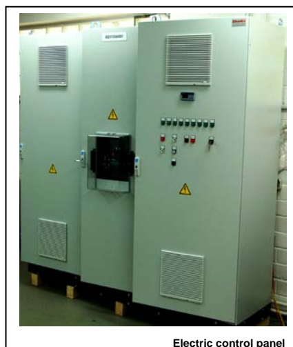
Electric control panel
